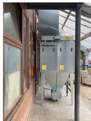
MCP-4-16SL Production Welding
